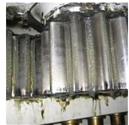
Open gear lubricated with Interflon Grease LS 1/2.
